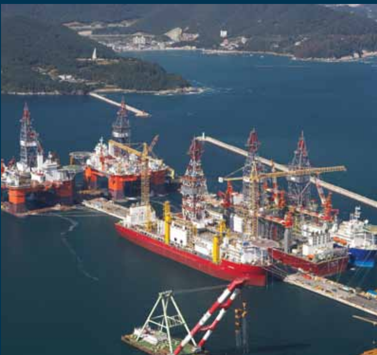
Semi submersibles and drillships, all with Aker Solutions' complete drilling packages installed
