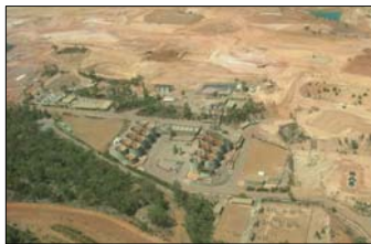
Boddington gold mine project, Australia
