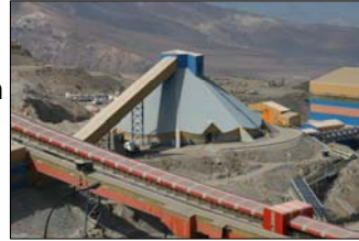
El Teniente project in Chile completed January 2007
