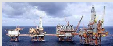
Valhall redevelopment steel structure Contract value: ~NOK 450 million
