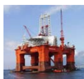
Drilling equipment & technology
