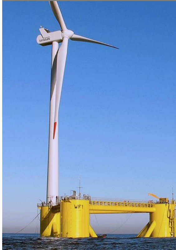
Proven deep-water foundation technologies
