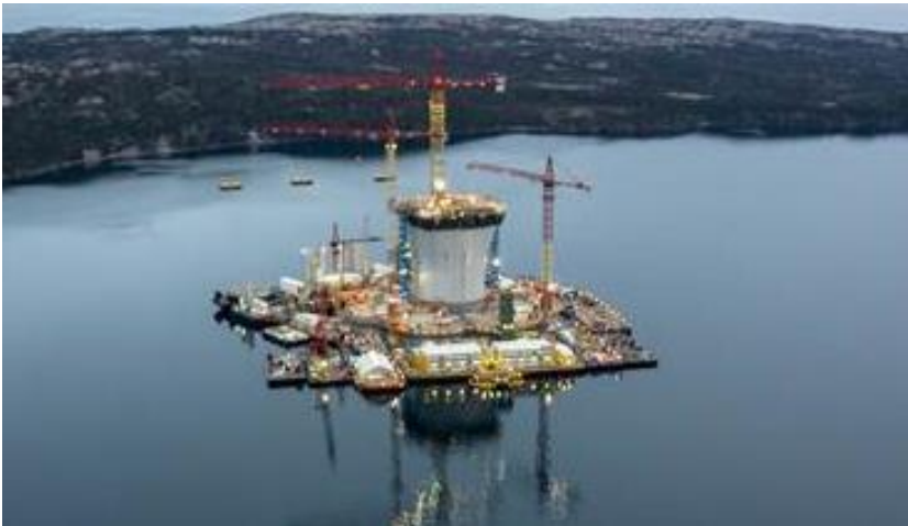
Hebron – Center shaft slip form completed
