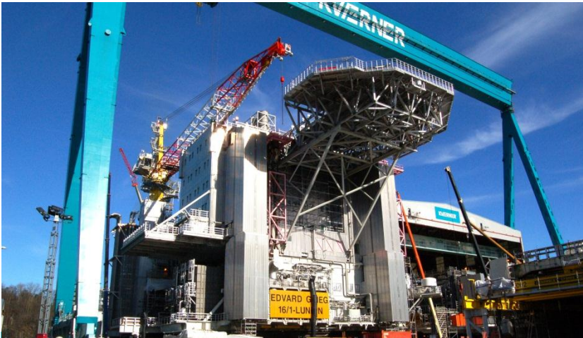
E. Grieg topside – To be delivered mid-April 2015
