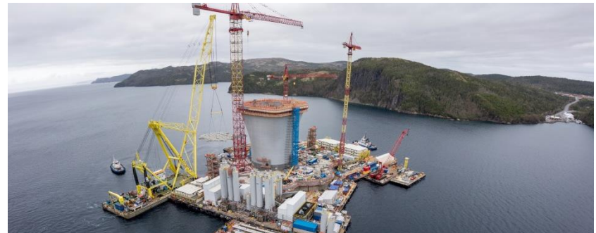
Hebron – Mechanical outfitting
