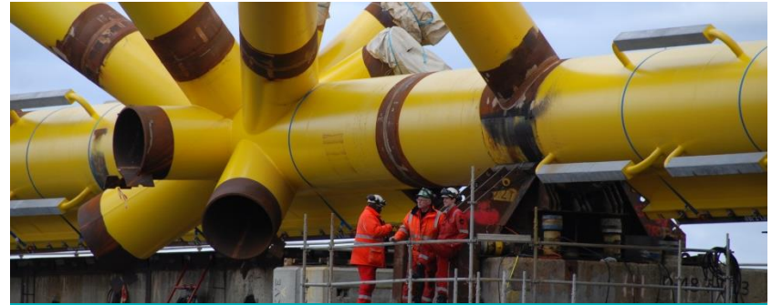
Sverdrup riser platform jacket roll-up
