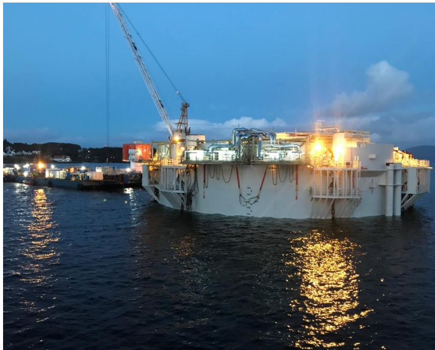
Aasta Hansteen spar during submergence test.
