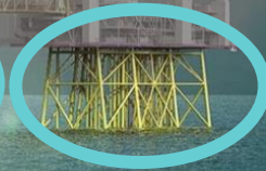
RP Riser Platform
