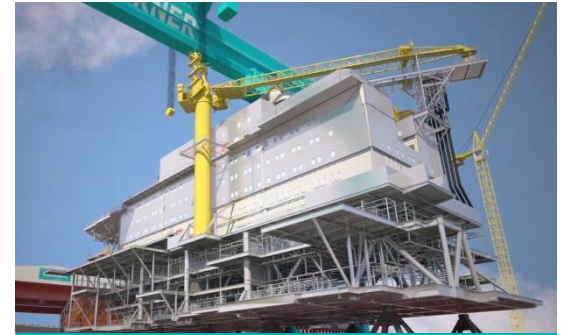
Johan Sverdrup Utility & LQ topside
