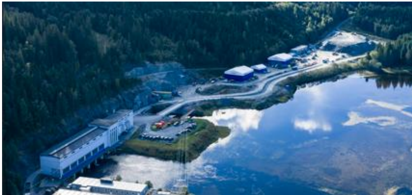
Svean Hydropower Plant
