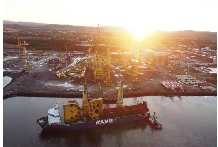
Major structures for Sverdrup riser platform jacket arrived in Verdal.
